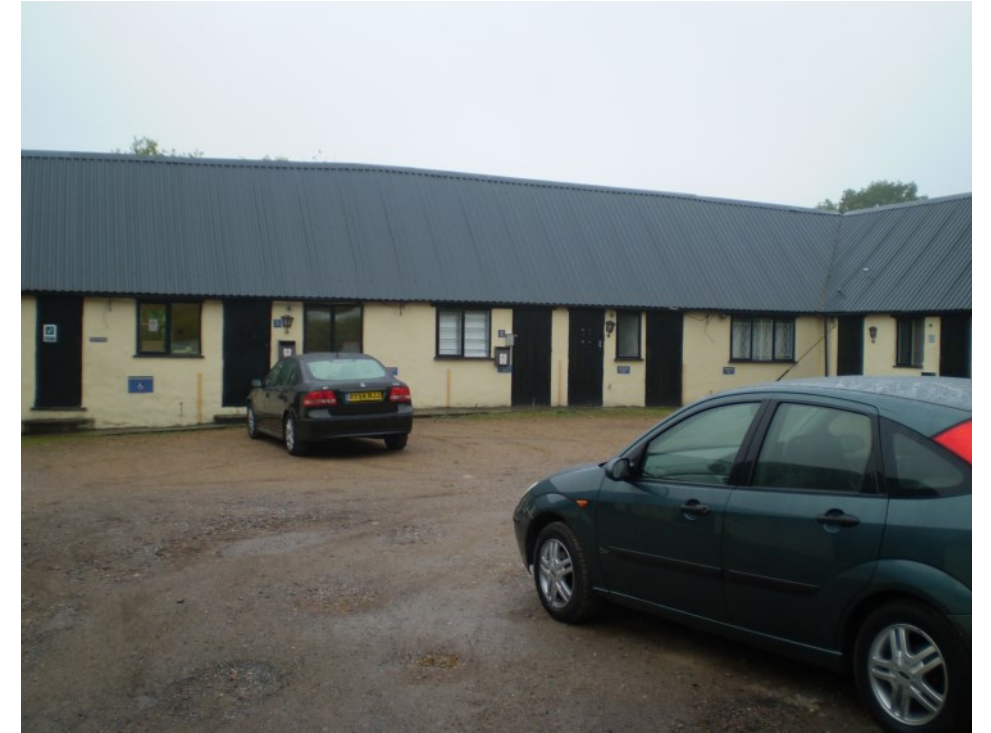
03 View of the commercial units and parking area
