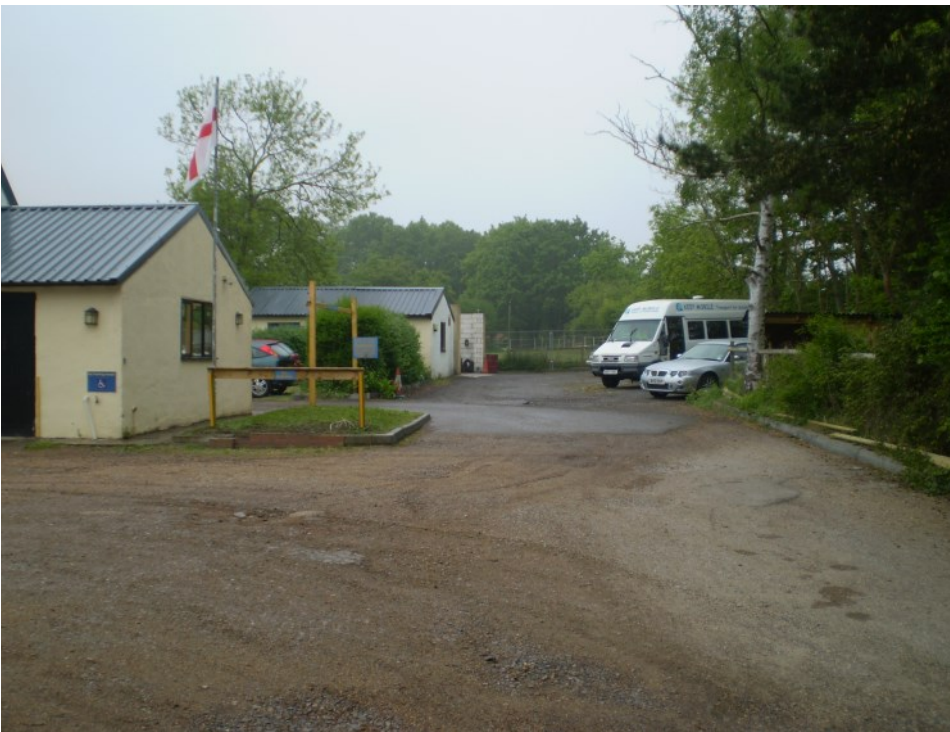
04 Extensive existing hardstanding, viewed from the site entrance
