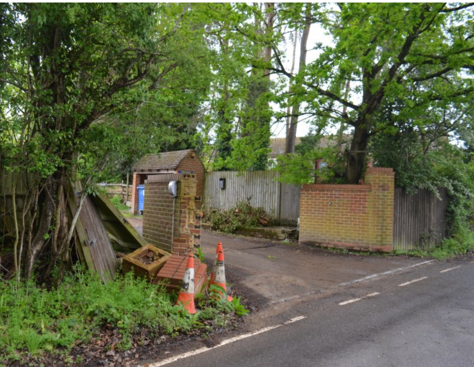
04 Existing site access from Evendons Lane, looking north-east
